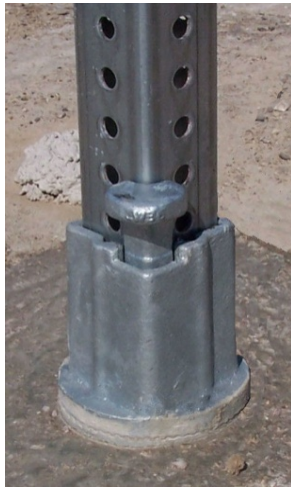
(Fig. 2) Stem Base Flush Mounted in Concrete
