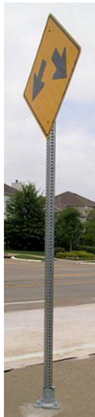
(Fig. 2) Stem Base Flush Mounted in Concrete
