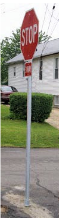
(Fig. 2) Stem Base Flush Mounted in Concrete
