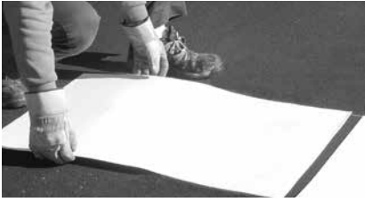
Clean the surface to remove any debris. Preheat the pavement surface to a minimum of 300° F.
