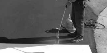
Heat HotTape™ with a propane heat torch such as the Magnum Heat Torch.
