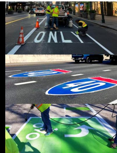
Tuff-Mark and Tuff-Mark with Tuff-Grip - **90 and 125mil** Preformed Thermoplastic Pavement Markings
