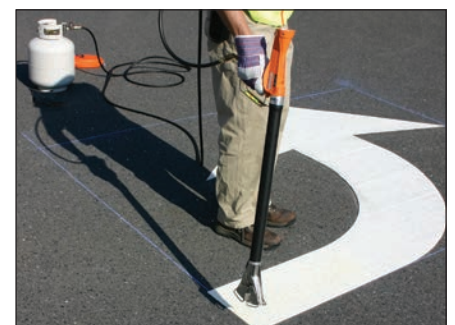
Multi-colored markings have interconnected material for ease of handling and application.
