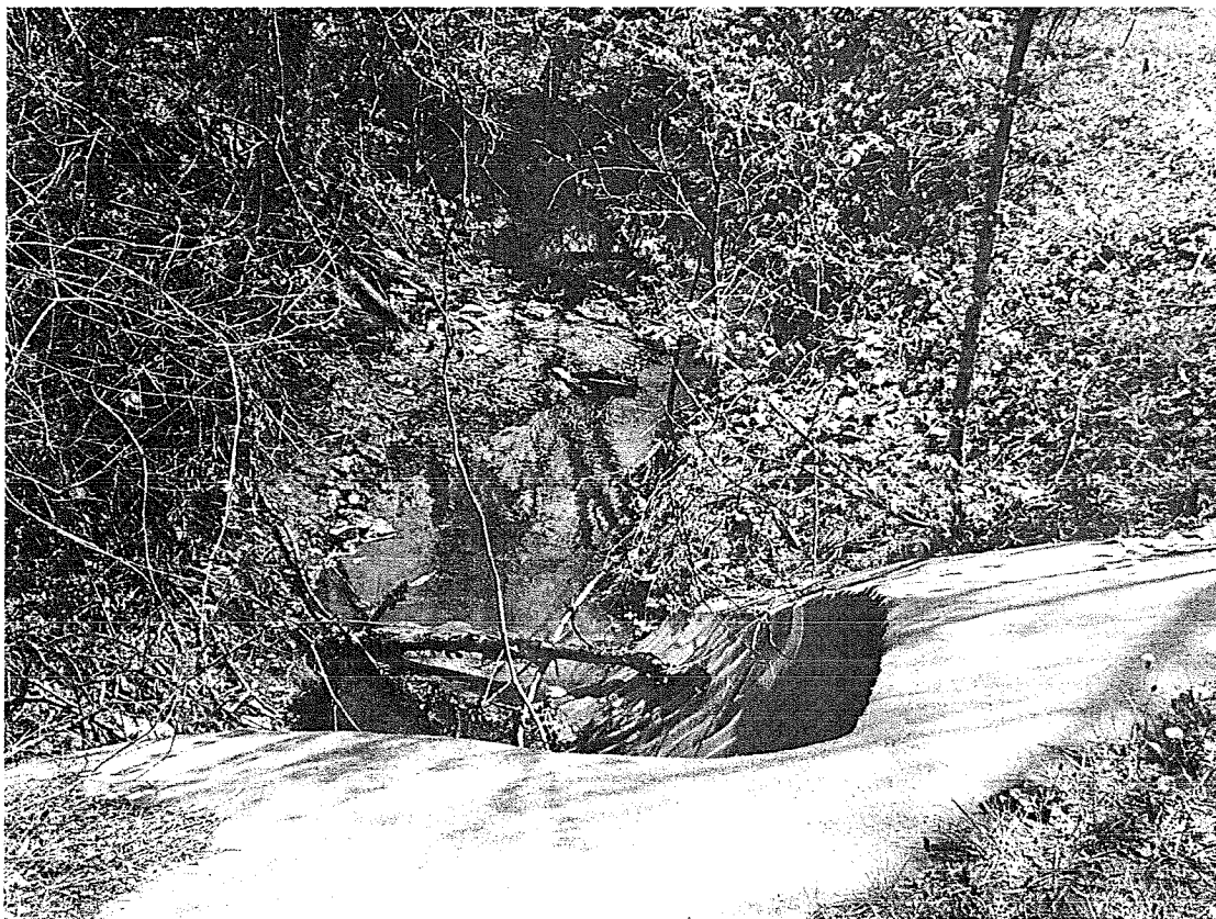
UPSTREAM end of 8.5' x 5.5' CMAP (~Sta. 110+12) looking Southeast
