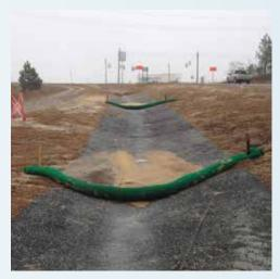
Check Dams: Use as a check dam device in stormwater ditches, channels, and swales on or near land disturbing activities.
