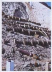
Courtesy Jenman Enterprise, Melrose, MA Coastline Protection at Cape Cod, MA with stacked & contoured 20" FibreLogs™ with double coir net.
