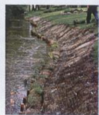
Courtesy Heartland Restoration, Ft. Wayne, IN 12" PlantLog™ days after installation (left) and after one year (right) along a legal drain in South Bend, IN.
