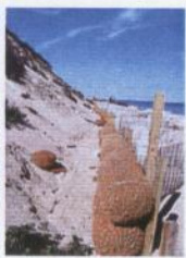
Courtesy Jenman Enterprise, Melrose, MA Coastline Protection at Cape Cod, MA with stacked & contoured 20" FibreLogs™ with double coir net.
