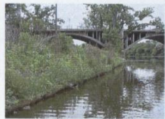
Courtesy Slusser's Greenthumb, Logansport, IN BankSaver System FibreLog™ performing along the St. Joseph River seven years after install.
