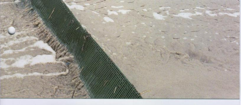
As water flows through the GeoRidge berm, its velocity and energy are reduced. As a result, silt and sediment are deposited upstream of the berm aiding in rediment control.
