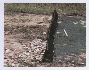
New vegetation growing on the downstream side of the GeoRidge. Note the significant sediment the berm has prevented from flowing downstream.
