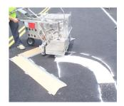
Thermoplastic Pavement Marking Compounds have been used extensively in the road marking industry since the 1950's as a durable and economical pavement marking on the world's highways. It remains today the durable marking of choice due to long term performance, cost benefit and a wide range of application techniques that improve motorist safety and provide agencies a long term marking solution.
